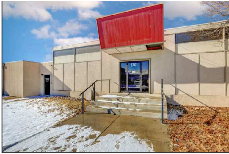
The buyer will complete renovations once a new tenant has been set.
